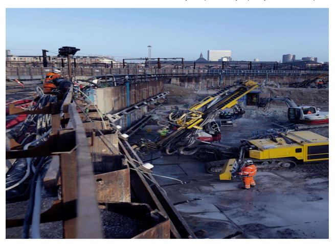
ment of a 100% reinfiltration of water, which was a challenge to handle in central Copenhagen. That is why we designed a cut-off effect to limit the infiow of water into the limestone deposits in the ground.
