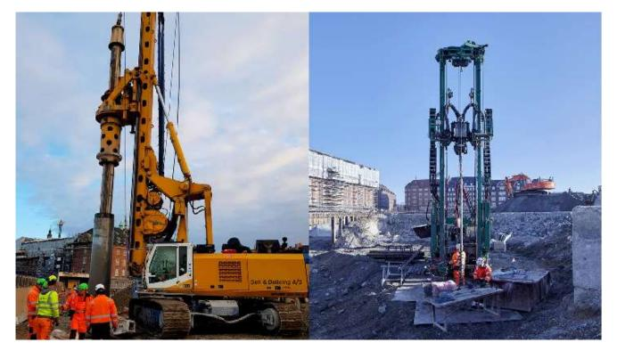
Furthermore, for Danske Bank's new headquarters, comprehensive piping works were performed using 2,500 driven concrete piles, 500 uplift anchors, 80 GEWI piles for crane foundations as well as 70 drilled piles in dimensions between DN880-DN1800 millimetres.
